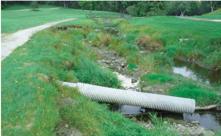
stream banks & toe of slope
